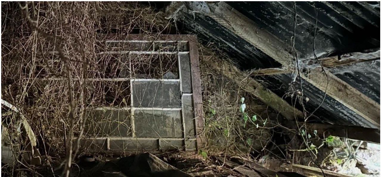
The original glass panelled door, still in the loft of the barn.
